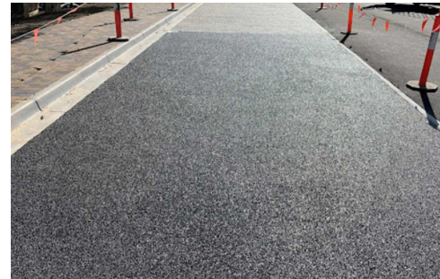
Porous asphalted pavement
